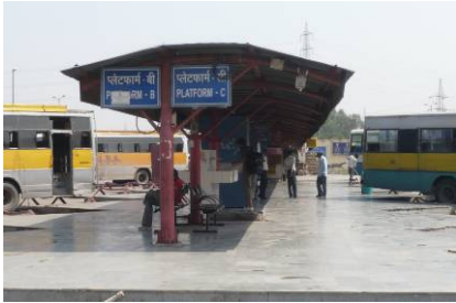
Platform and Passenger Shelter
